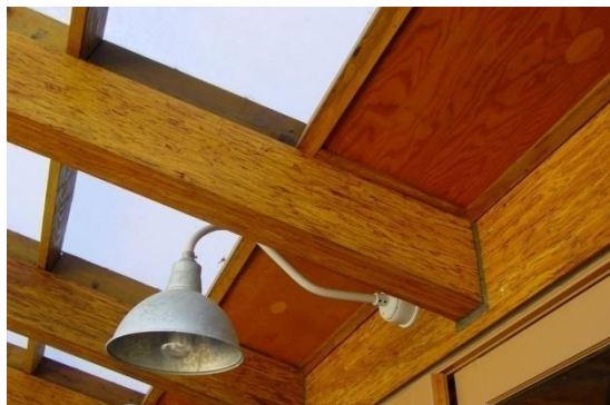
Example assembly of Micro-Lam Timber Framing.
