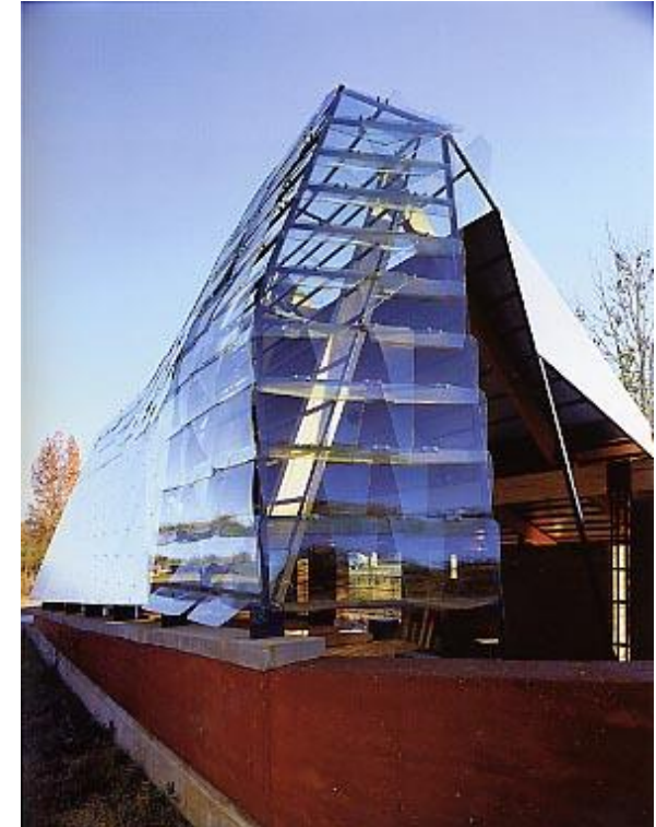
An example of recycled materials in a small open air community building in rural Alabama.
