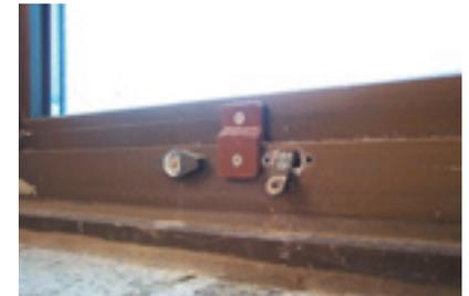
**Figure 13.2.** All operable windows on the north facade have been bolted shut.
