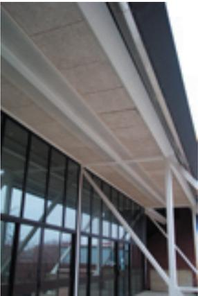
**Figure 18.2.** Top and bottom louvers are "closed."
