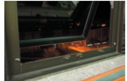
**Figure 17.3.** Operable windows on the north facade are open.
