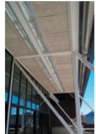
Figure 19.2. Top and bottom louvers are "open."
