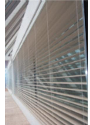
Figure 19.1. Blinds are in the "filtered" position (horizontal).
