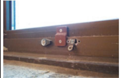
**Figure 9.1.** Permanently locked studio window.
