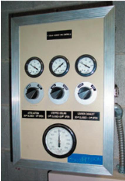
Figure 26.1. Louver control panel.
