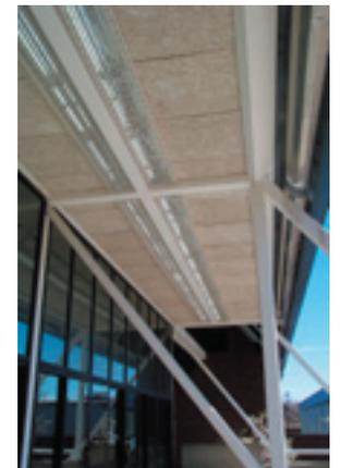
Figure 23.2. Top and bottom louvers are "open."
