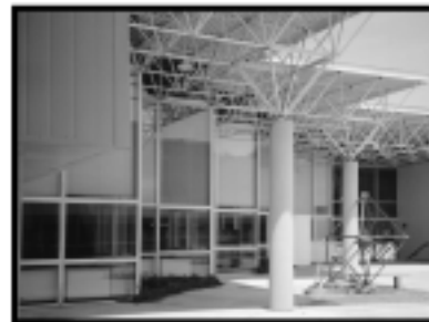
Figure F.2b : Wall Between Library and Community Concourse, Exterior
