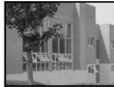
Figure C.3a : North Window, Exterior
