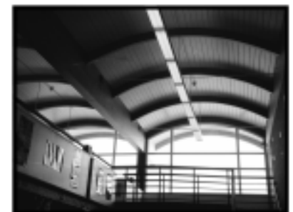
Figure P.5c : Interior View: North Window and Ceiling Fixtures
