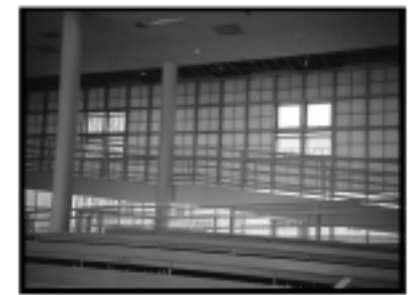
Figure C.4b : South Wall, Interior
