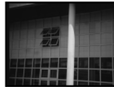
Figure C.4a : South Wall, Exterior
