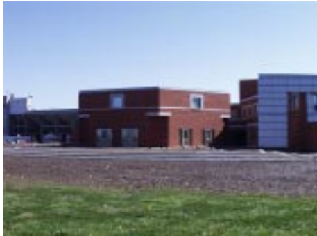
4. South view of building.
