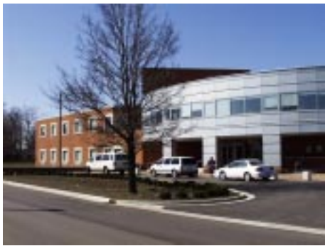
1. View of main entry from the east.
