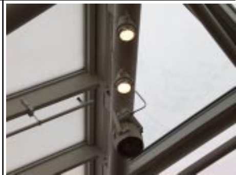
12. Detail of spotlights in conservatory.
