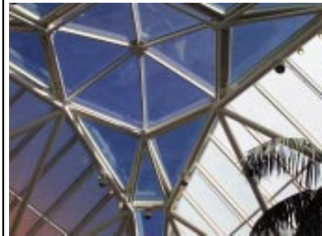
41. View of skylight in conservatory.
