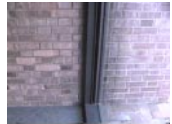
Figure 5 Fixed glazing mullion with integral air supply/air return channel.
