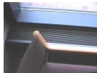
Figure 13 View of the baseboard convactor units located below the north-facing glass of the addition.
