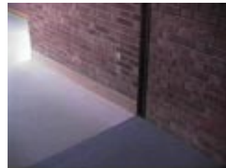
Figure 12 View of the diffuser cover placed over the original mullion location at the Galleria connection to the main library space in the original building.
