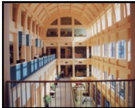
Fig. 46-b The Office Wing atrium as it is, showing a much cooler space with a lower material reflectance that can reduce the harsh effects of bright direct beam radiation.
