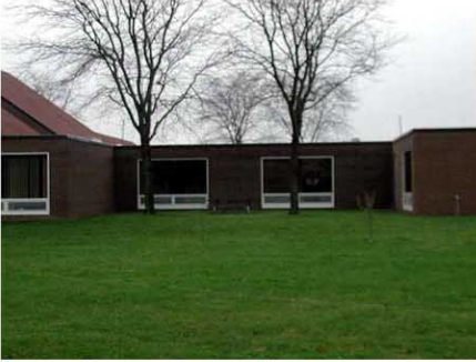
Fig. 7A: A view of the classroom windows
