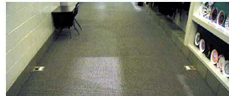
Figure 10C: Photograph showing placement of one group of Stow-Away's.
