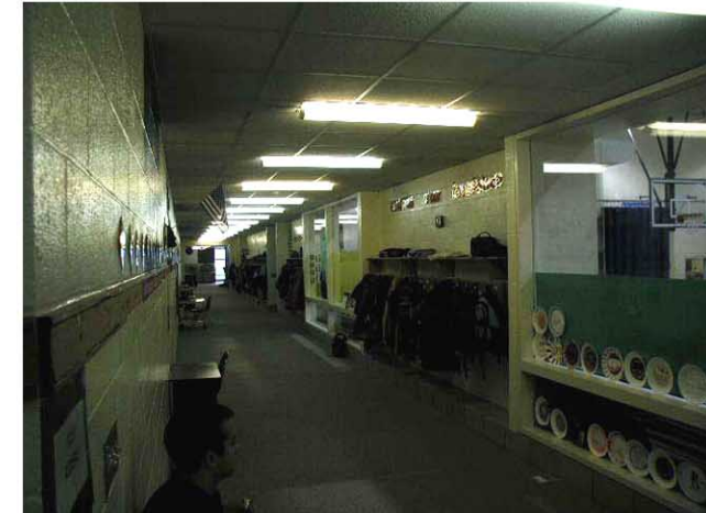
Fig. 9B: Photograph of the corridor, showing the large windows of the gymnasium and exterior window.
