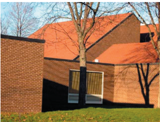
Fig 1.2, 1.3 - View of roof monitors with clerestory windows. Note: images show the roof structure over the art room.
