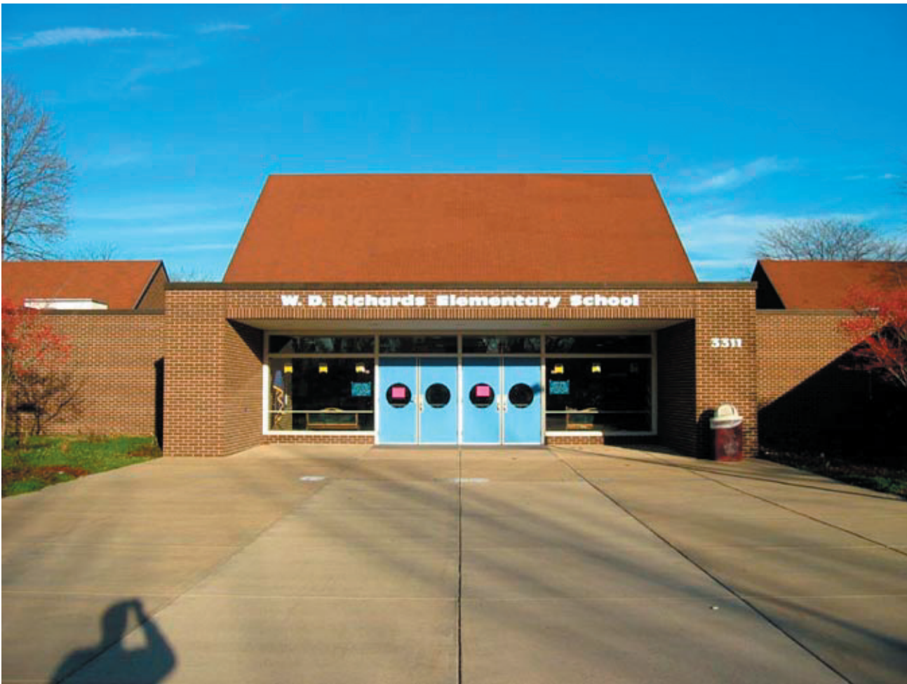
Fig 1.1 - W. D. Richards Elementary School main entrance
