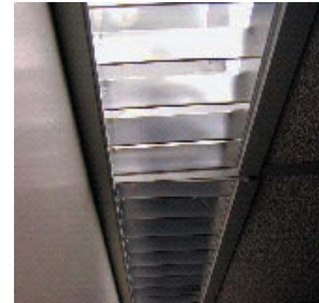
FIG.3.2 34 W, T12 Rapid Start SUPER SAVER fluorescent lamp, Cool White phosphor, 4200K color temperature, 62 CRI, SAFE-LINE coated
