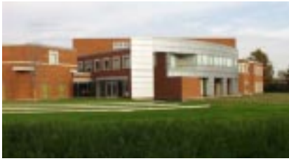
Fig. 1 Exterior photograph of the Alumni Center taken from the Southwest corner
