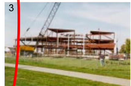
Figures 1-3 show the Alumni Center under construction
