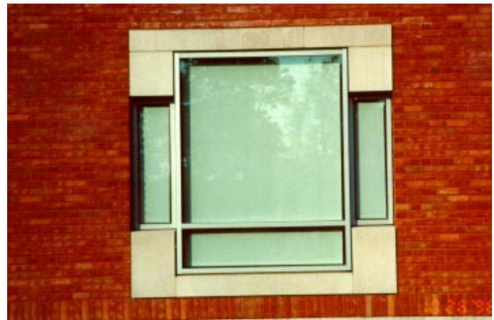
Fig. 4 exterior window of library showing: sunshades relative size of shades to window
