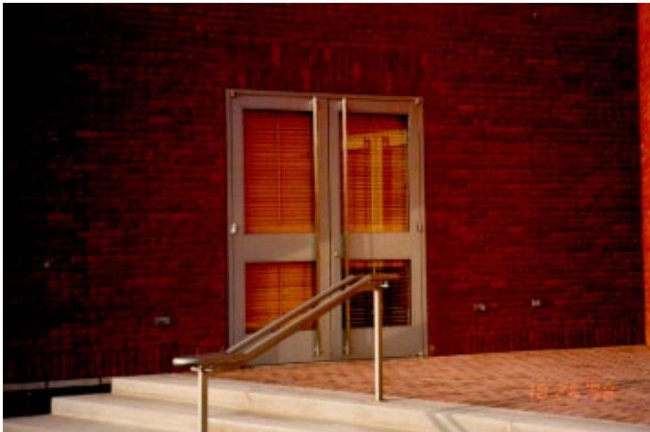
Fig. 3 one of two typical exterior doors showing: louvres opportunity for daylight
